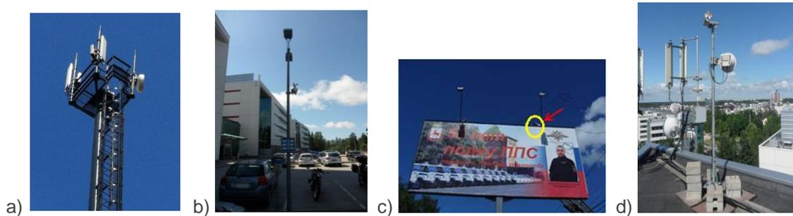
Figure 49: Typical small-cell sites a) telecommunication mast, b) lamp pole, c) billboard and d) rooftop BTS site.
