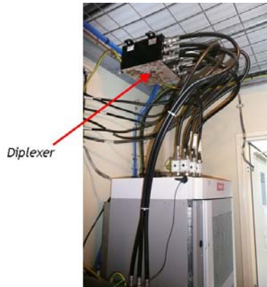
Figure A.13.44: Diplexer multiplexing UMTS and DVB-SH signals
