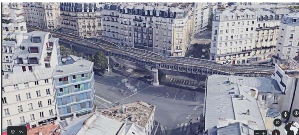
**Figure 5: Metro Line 6 of Paris on a viaduct with parallel road and crossing road
