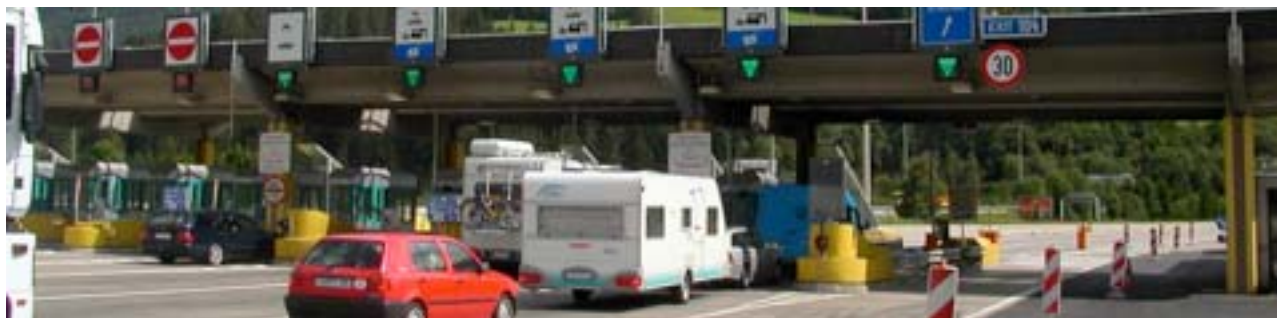
Figure D.3: Typical toll plaza with an automatic barrier (left) and automatic lanes (right)
