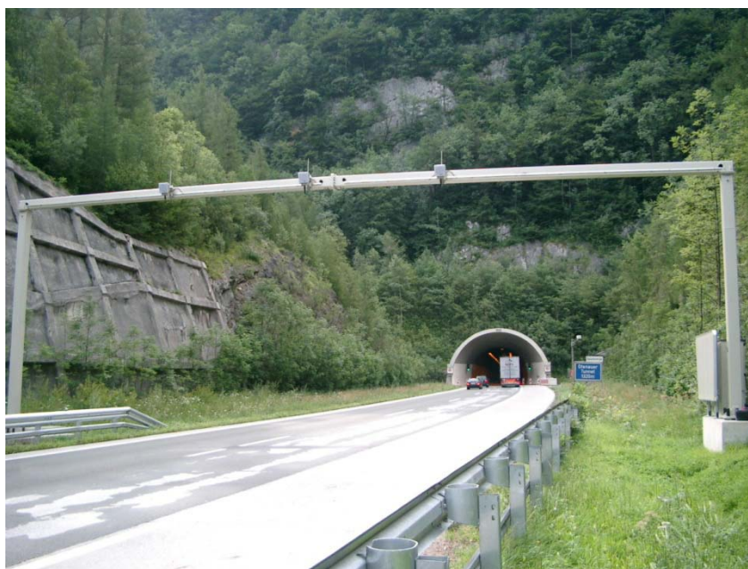
Figure 2: Typical free-flow installation with three lanes
