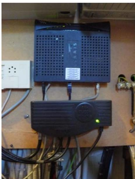
**Figure 10: In-home set-up with NIU and cable modem**
