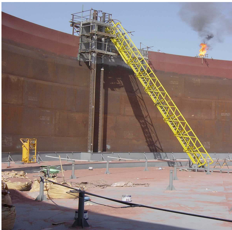
Figure 4: Typical EFRT with perforated still pipe under construction
