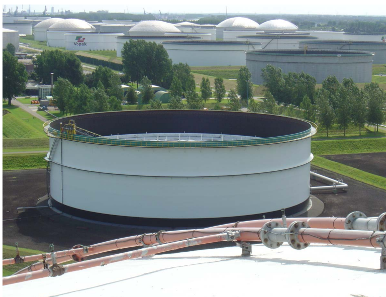
Figure 2: Example of an external floating roof tank with still pipe and TLPR
