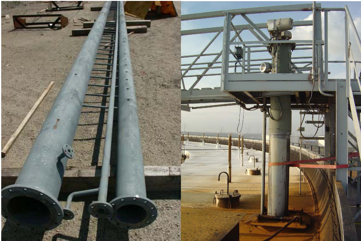
Figure 3: The perforated still pipes ready for installation in EFRT (left); operational perforated still pipe with floating roof (right)
