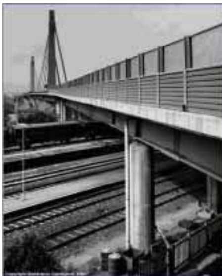
Figure B.6: Bridge view - 206 m length
