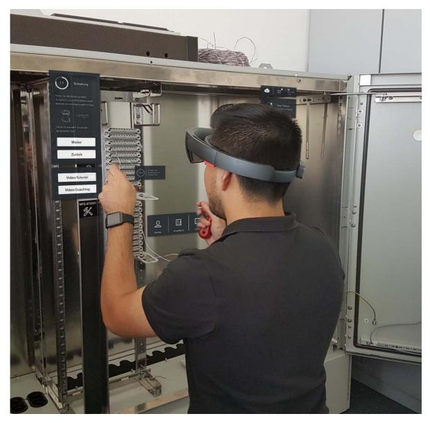
Figure 5: Wiring in a street cabinet
