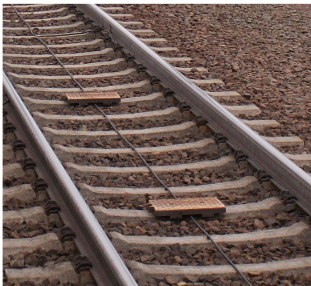
Figure 4: Eurobalise installed in the middle of a track (source: de.wikipedia.de)
