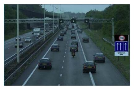
Figure B.10: Hard shoulder in use as a running lane, Netherlands (courtesy of Rijkswaterstaat)
