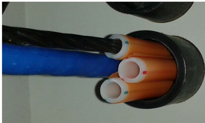
Figure 9: Installation of sub-ducts to provide segregation
