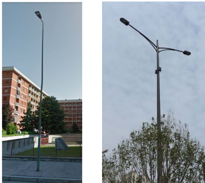
Figure C.3: Example of Lamp-posts not allowing mounting RRUs on top position
