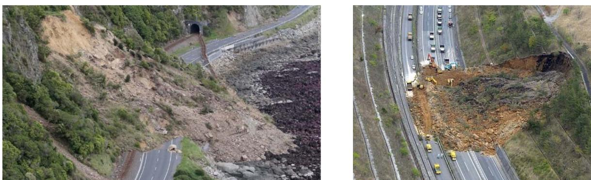
**Figure A.10: Cut slope failure examples**
