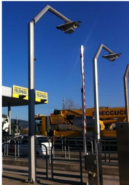
**Figure 3: Typical HDR-DSRC RSU installation**
