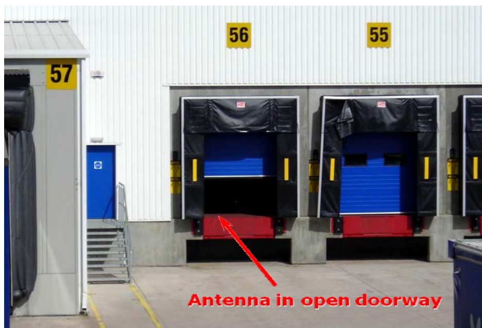
Figure C.3: Location of RFID Antenna
