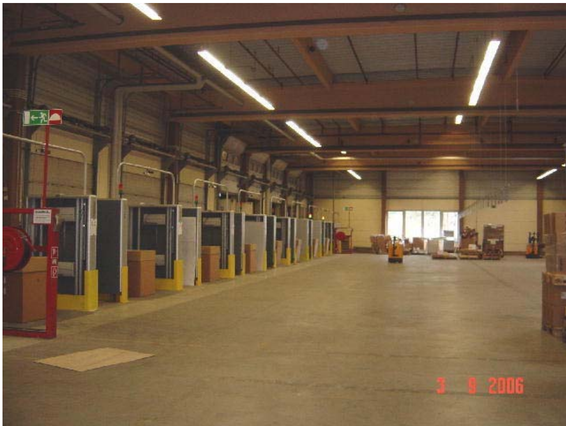
Figure C.1: Portals at dock doors on the left hand side of the photo inside a distribution centre
