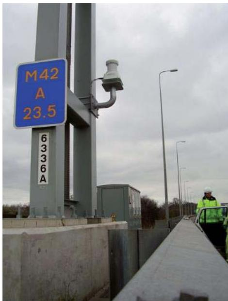
**Figure B.11: Radar installed for all lane incident detection in the UK**
