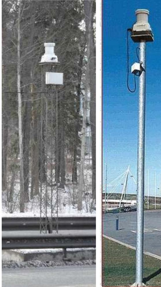
**Figure C.3: Radar mounting posts**
