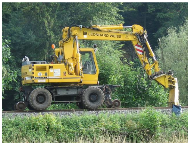
Figure A.2.1.1.4: Typical track area work situation
