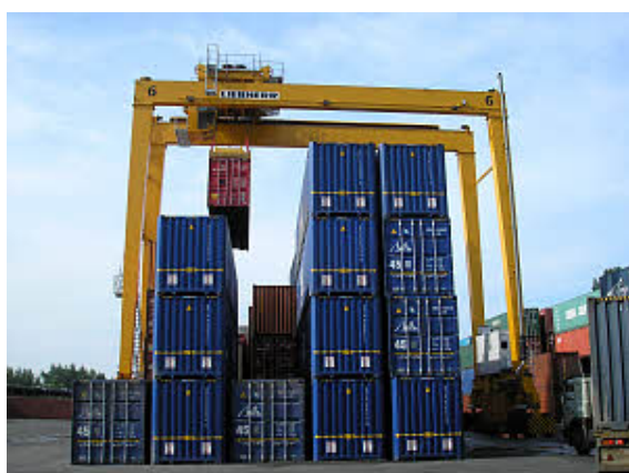
Figure A.4.1.5: Crane for container
