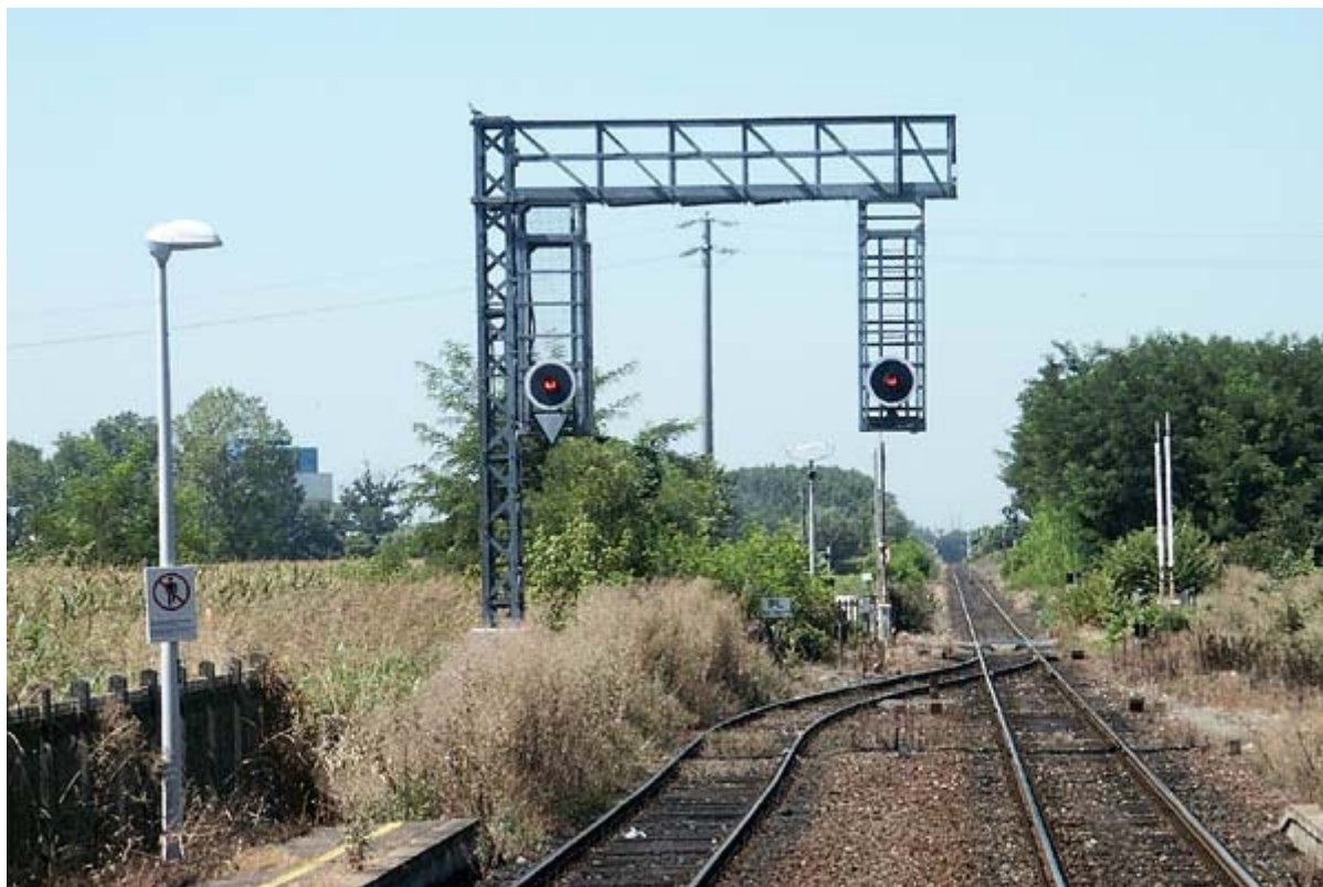
Figure 7: Typical railway signal
